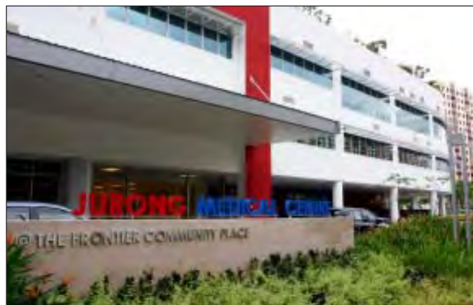
Jurong Medical Centre is situated in a three-storey stand-alone facility.
